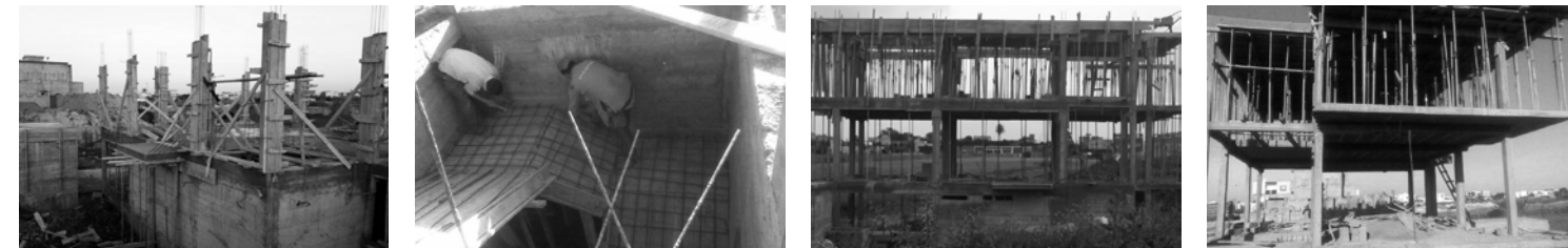
Construction site - Contract administration and field review
